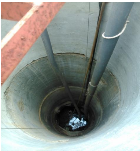
Fig 1 Well of Power house at site
