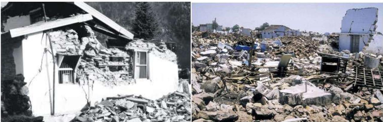
**Figure 1: Damage to stone masonry houses and Collapse of the housing colony at Gawana**
