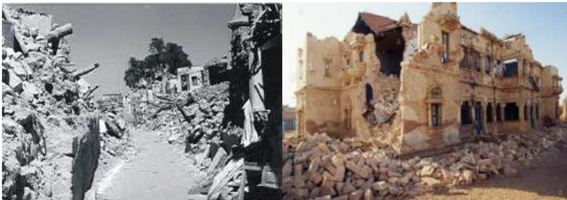
**Figure 2: Damage to stone masonry houses and Collapse of two storey stone masonry building Bachau**
