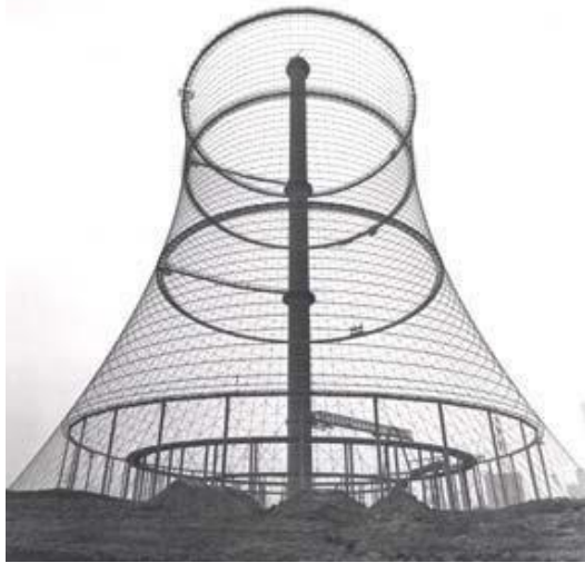
Figure 1 Cooling tower Schmehausen
