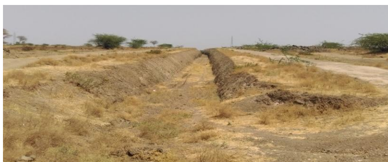
Figure 1: Under construction of NLBKBC
