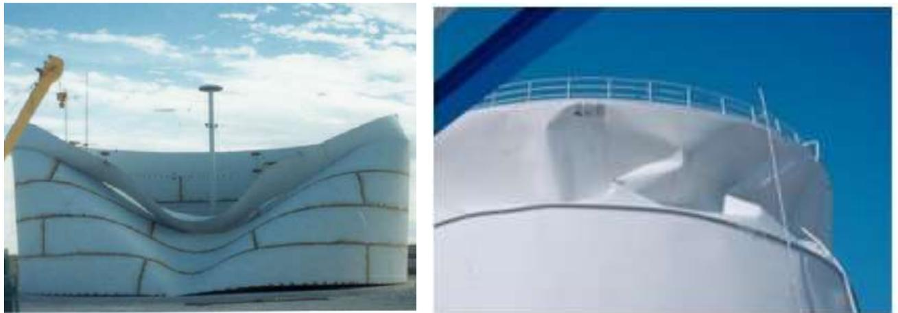
a) Roof and shell buckling
