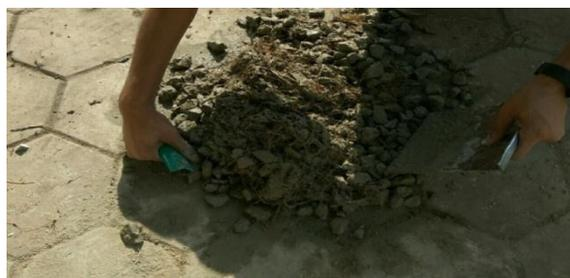
Fig2.2:- mixed with coconut fibre
