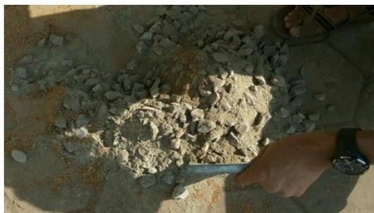
Fig2.1:- mixing of cement and aggregates
