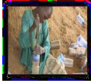
Fig. 5 Method of filling the plastic bottles for using in the building.
