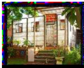
Fig. 7 Green building built using plastic bottles.
