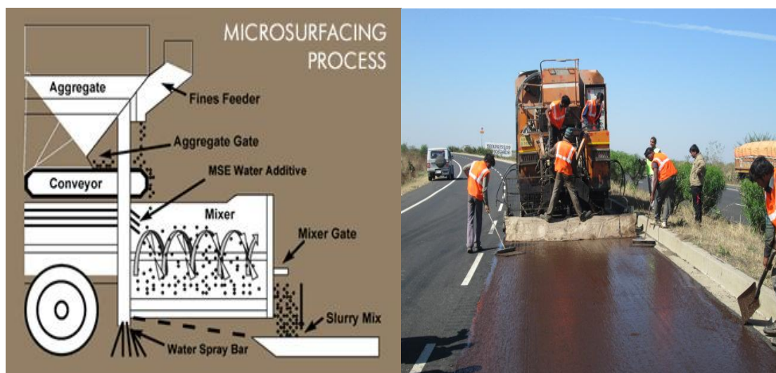
Figure 1. Micro surfacing Process Figure 2: Micro Surfacing
