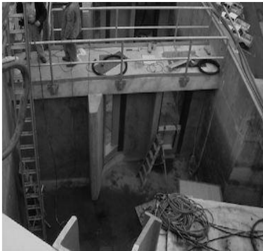
Fig. 1 GFRP Ice Harbor lock and dam fish weir
