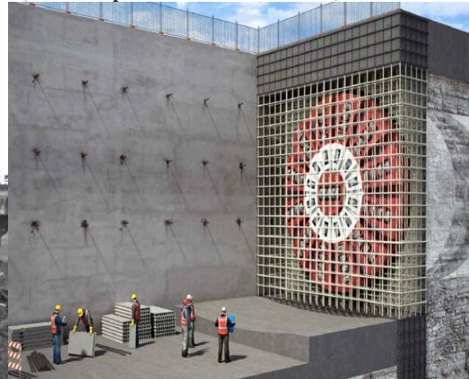
Fig. 6 GFRP soft-eyes for tunnel excavation
