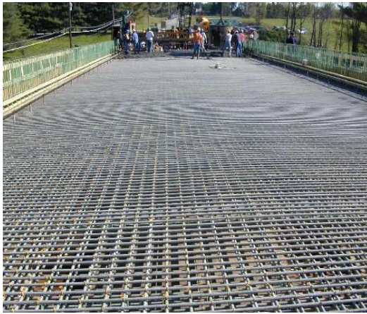
Fig. 3 GFRP reinforced-concrete bridge deck (Morristown, Vermont)
