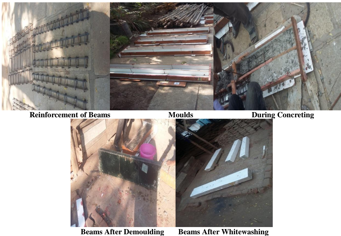
Plate 1: Photos of casting of geopolymer Beams
