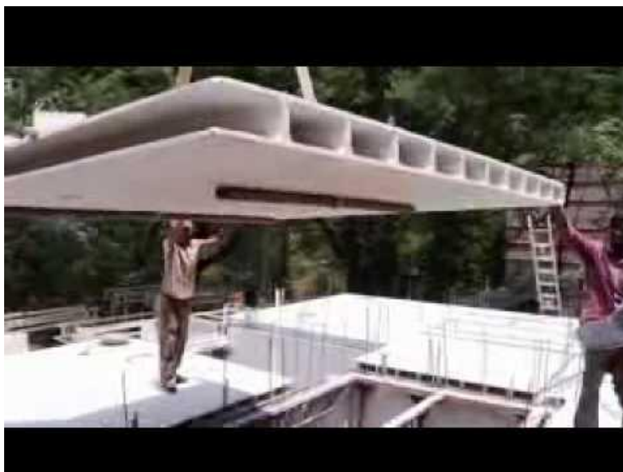
Figure. 1: Glass Fiber Reinforced Gypsum Panel
