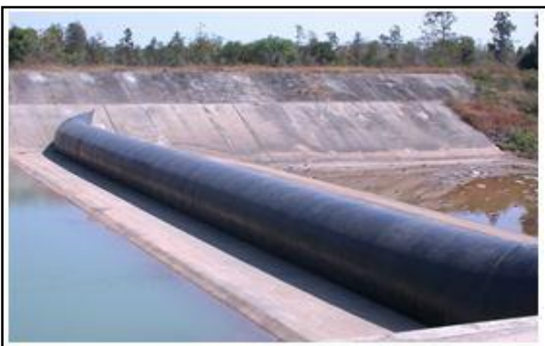
Figure 5- Inflated Rubber Dam in Irrigation Canal
